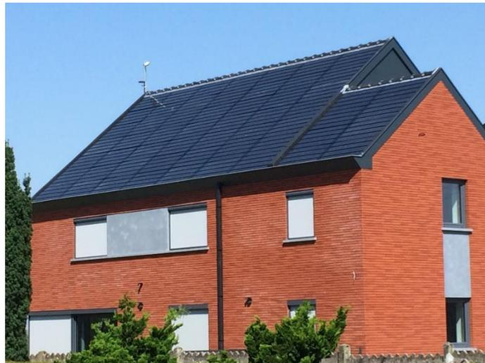
Figure 3. The 57 RS modules on the roof of the demonstration building.
