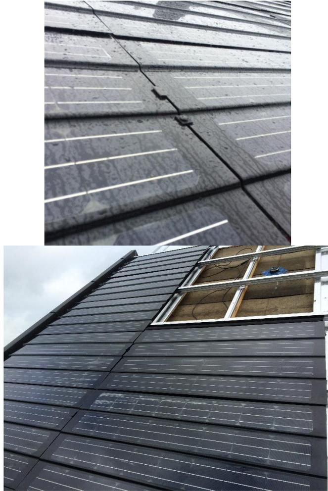
*Figure 4. RS modules overlap, without connections in between the panels (left picture), and the gutter between the panels to collect the rain (right picture).*
