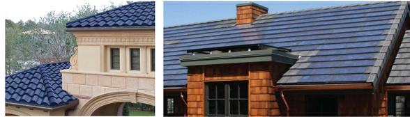
Fig.1. Examples of BIPV tiles on building roofs, Solar Thermal Magazine (left) (2010) and Applied Solar (right) (2010).
