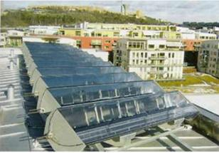
CPC Hybrid PV/T – WATER solar collectors
