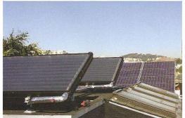
PV/T collectors can be applied to buildings, instead of separate solar thermal and photovoltaics
