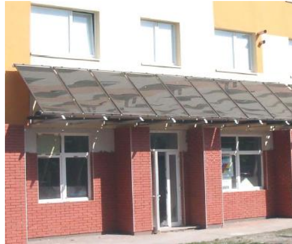
Flat STC are preferable for overhangs as they can protect from rain and snow.
