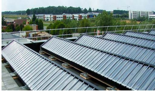
SolarDuct is a solar heating system that heats ventilation air before it enters the air handling units. The system uses an all-metal collector panel (transpired solar collector). Perforations in the panels allow the heat that normally collects on a dark surface to be uniformly drawn through the SolarDuct panel and then ducted into the conventional HVAC system.
