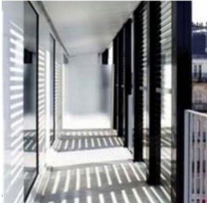
Semitransparent collector encapsulated into a double skin facade, Social housing, Paris, France, www.iea-shc.org
