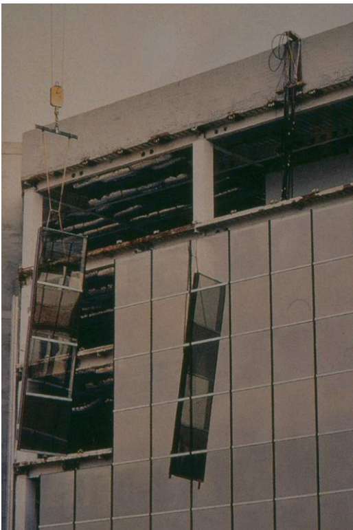
Hybrid Photovoltaic/Thermal facade constructed of prefabricated glass modules.
