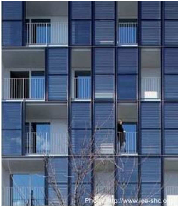
Semitransparent collector encapsulated into a double skin facade, Social housing, Paris, France, www.iea-shc.org
