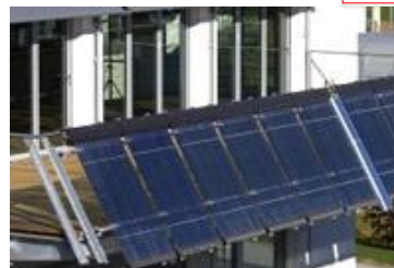
For balcony railings construction both types are suitable, but vacuum tubes enable better view of the surroundings.
