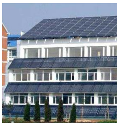
STC as shading device
