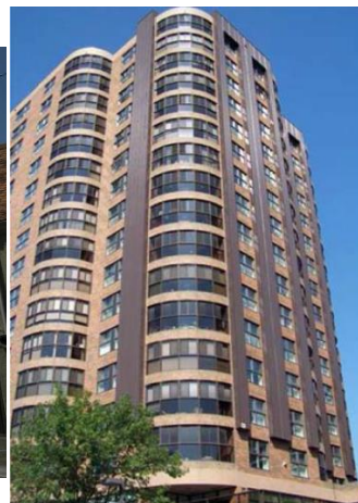
Residential building refurbishment, Fred Douglas Place, Manitoba, Canada SolarWall System
