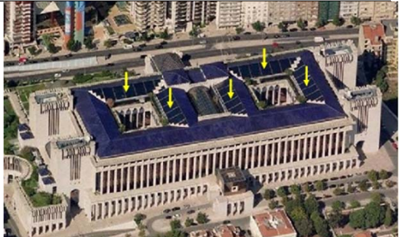
Fig.2: Integration of STC in a pitched roof (Caixa Geral de Depósitos, bank headquarters, Lisboa)
