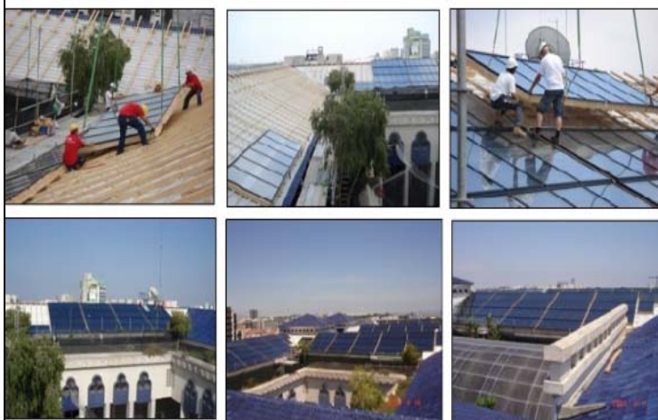
Fig.4: Installation of the STC in the roof
