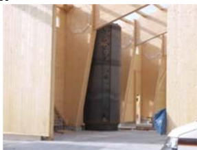
Floor heating under construction / Solar storage tank 17.000 l / Structure of the floor plate
