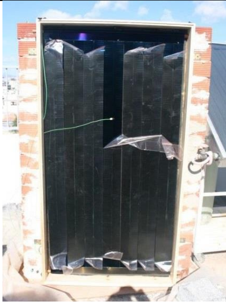
Figure 4.3. Positioning the ready-made absorbing plate in the integrated hot water collector
