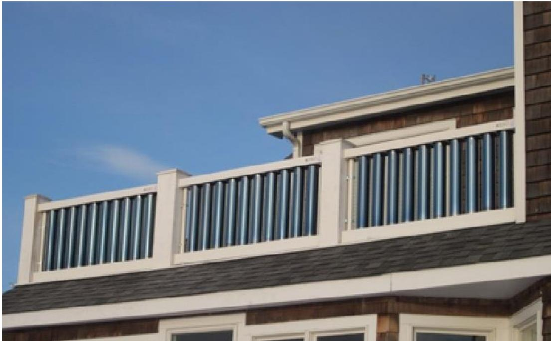
*Figure 2.18 The JET Solar Fence (JSF) installed in a domestic building in USA.*
