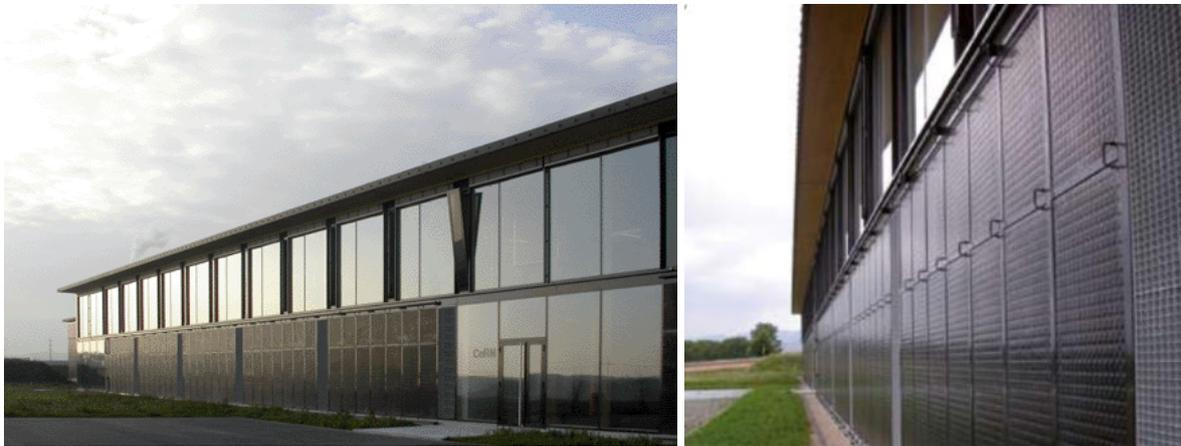
*Figure 2.17 The BISTS integrated onto the façade of the Centre d'entretien des Routes Nationales (CeRN) in Switzerland.*
