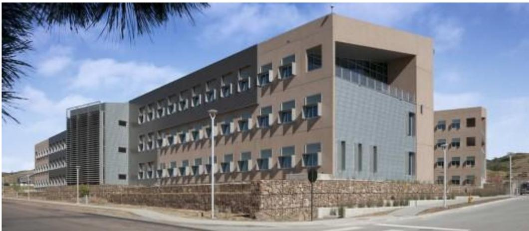
*Figure 3.9 RSF building in Colorado: SolarWall façades.*
