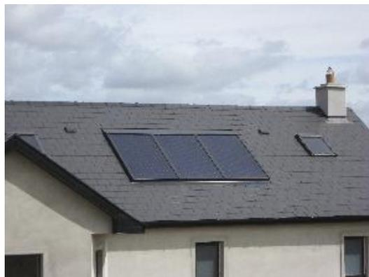
*Figure 2.16 The Integra In-roof Integrated Solar Collector installed onto the roof of a new domestic dwelling in Ireland.*
