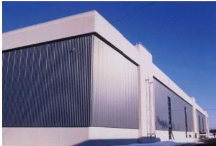
*Figure 3.8 The SolarWall BIST in the Canadair industrial facility in Montreal, Canada.*
