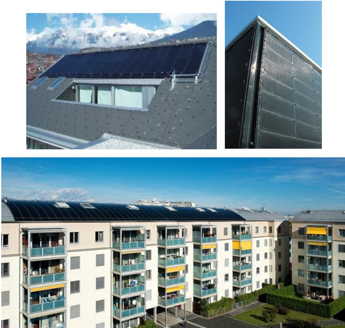
*Figure 2.5 Examples of the Energie Solaire solar collector as a BISTS on different types of buildings.*
