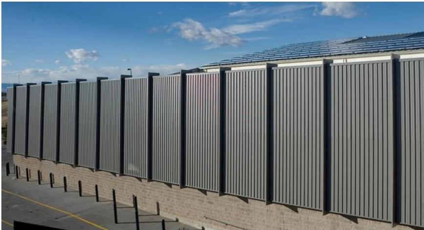
*Figure 3.18 The SolarWall installation on the Supercentre commercial building in Colorado, USA.*
