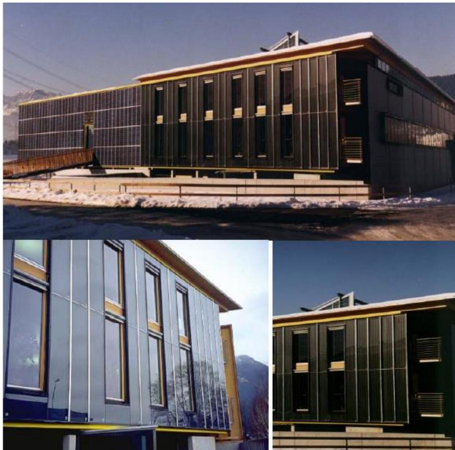
Figure 6.3 Solar integrated system in the AKS DOMA Solartechnik building in Austria.
