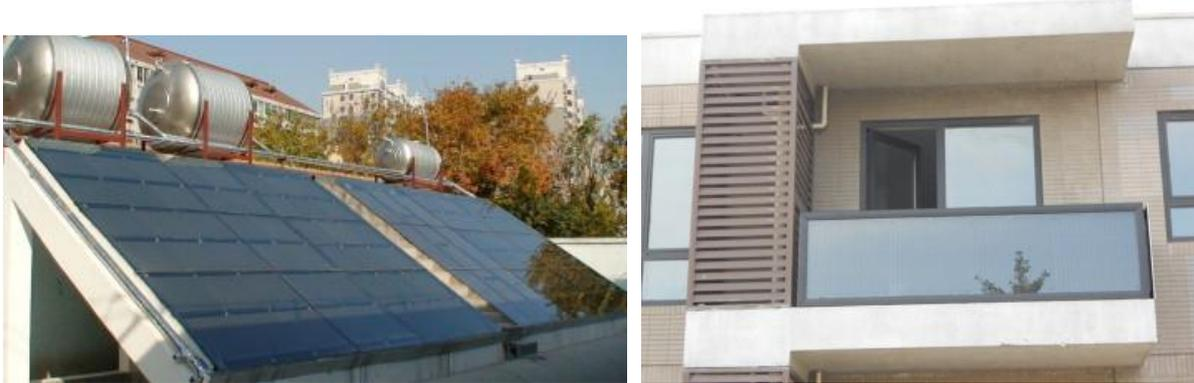
Figure 2.12 The all ceramic collector as a roof integrated system (left) and integrated as a balcony balustrade (right).
