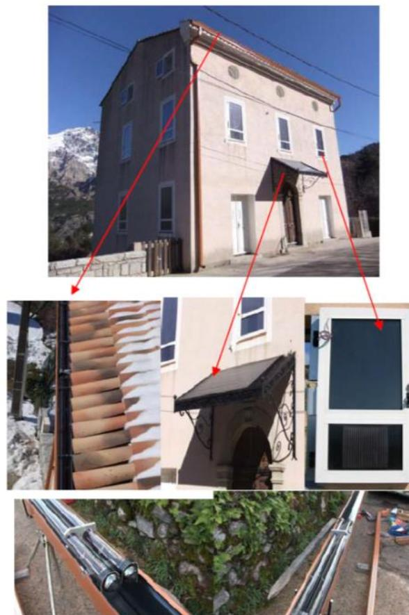
Figure 6.9 Combined BISTS application in Corsica.
