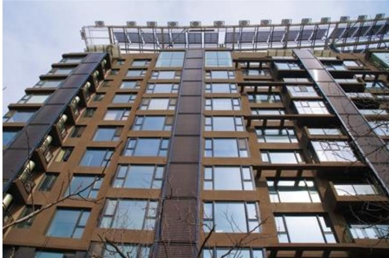
*Figure 2.19 Evacuated tube solar thermal collectors horizontally integrated onto the façade of a building in the 'Garden Utopia' Project in the Chinese city of Dezhou.*
