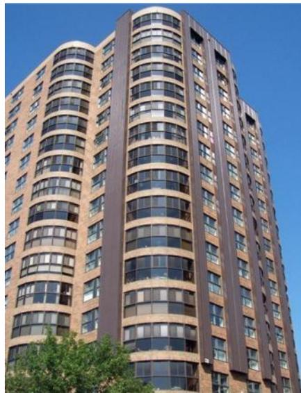
*Figure 3.14 The SolarWall installation on the Fred Douglas Place multi-residential building, in Manitoba, Canada.*
