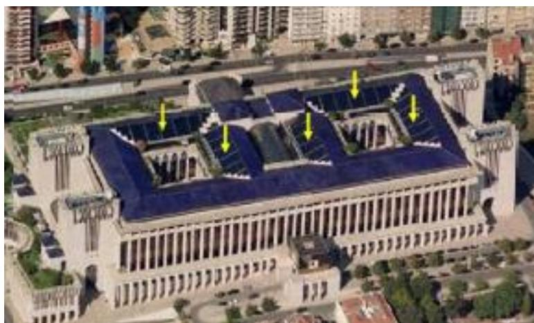
Figure 6.2 Integration of STC in pitched roof.
