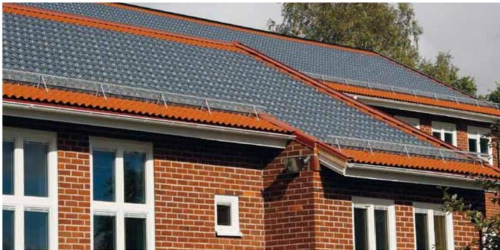
Figure 2.7 The Soltech Sigma Smart Roof solar collector integrated on a domestic building roof.
