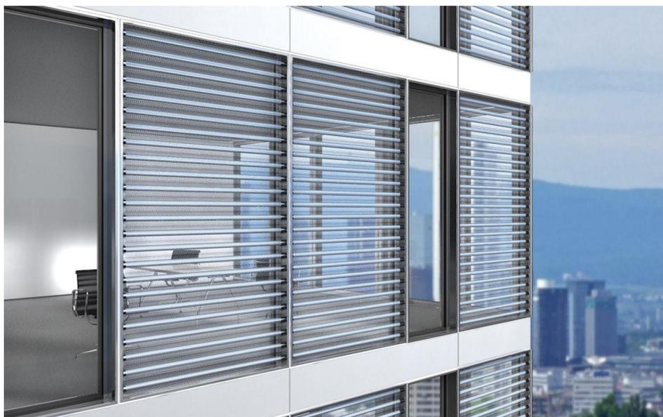
*Figure 2.9 The of University of Stuttgart BISTS on a building façade.*
