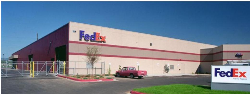
*Figure 3.13 The SolarWall on the FedEx building in Colorado, USA.*
