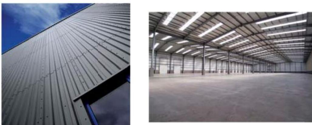
Figure 3.6 The Kingspan ISAC on the façade of a commercial building in Doncaster, UK.
