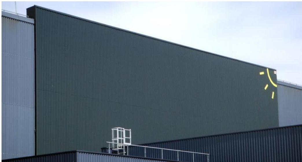
*Figure 2. Toyota Motor Manufacturing SolarWall system.*
