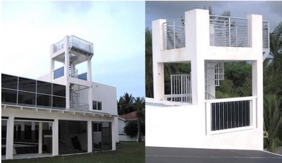
*Figure 2.15 GLE solar evacuated tubes in residential building in Florida.*
