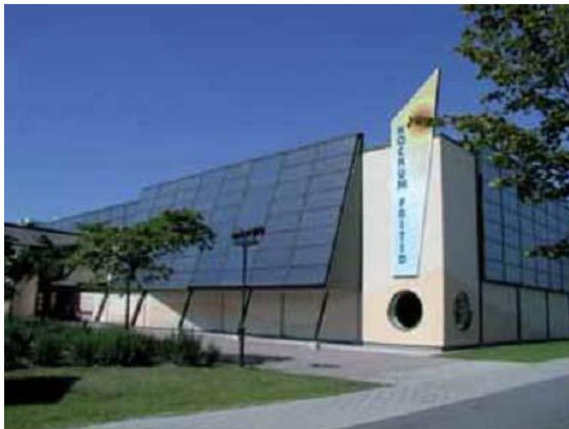
*Figure 14 Façade integrated collectors at Kockum Fritid in Malmo.*
