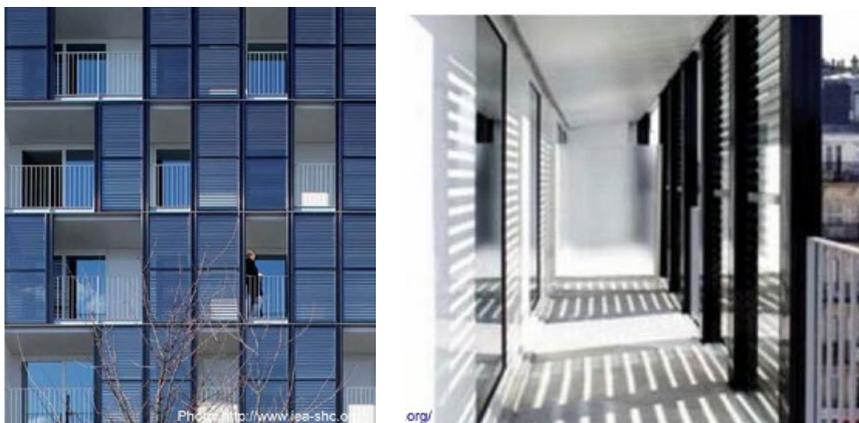
Figure 4.6. Semi-transparent collector encapsulated into a double skin façade, Social housing, Paris, France.
