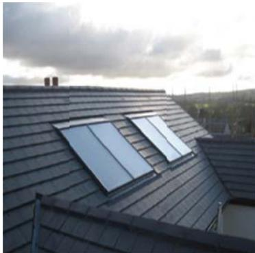
Figure 2.4. Roof integrated flat plate BISTS
