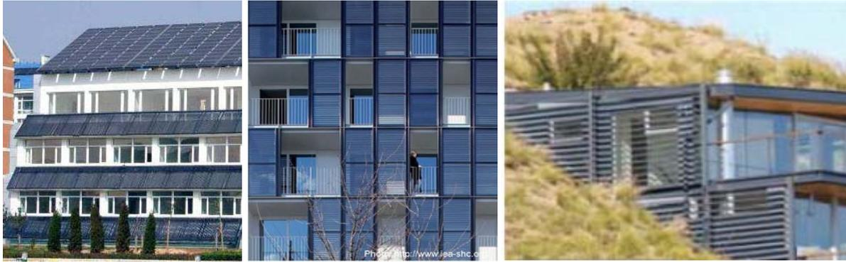
Figure 4.14. Solar thermal collector as shading device
