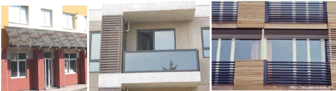
Figure 4.15. Solar thermal overhang and balcony railing
