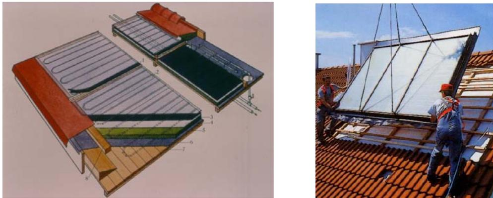
Figure 4.11. Roof integrated solar thermal collectors.
