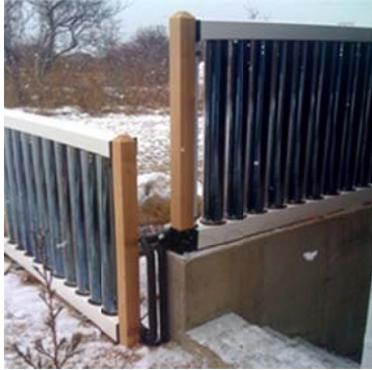
Figure 2.6. BISTS balustrade/railing feature
