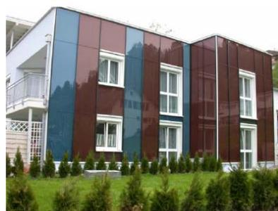
Figure 4.8. Glazed solar thermal integrated façades, appearance of suspended façade (curtain wall).
