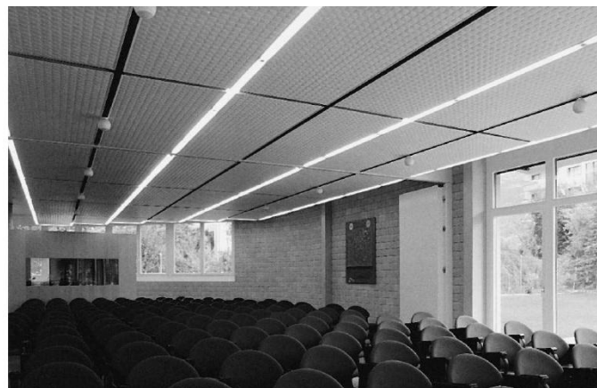
Figure 8.3 Heating and cooling ceiling in a meeting room.
