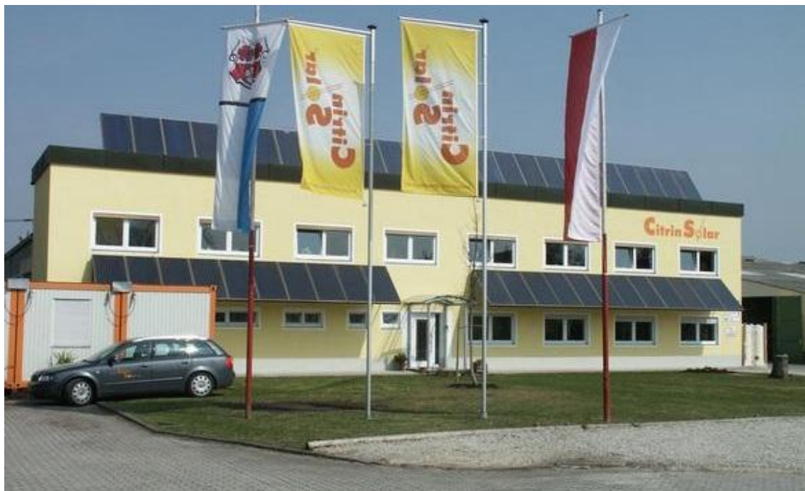
Figure 2.10 Roof and facade BISTS on the Citrin Solar factory (Germany).
