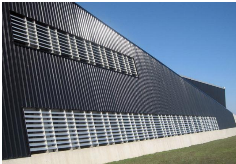
Figure 3.15 Greater Toronto Airport Authority – SolarWall system.
