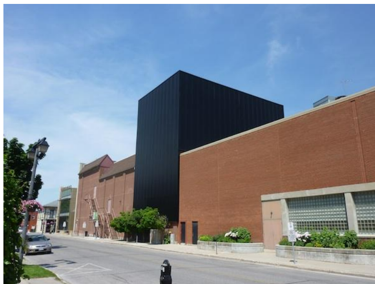
Figure 3.10 The SolarWall BIST in the Avon theatre building, Ontario, Canada.
