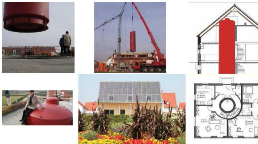
Figure 8.6 Solar water tank integrated in a solar building in Regensburg.
