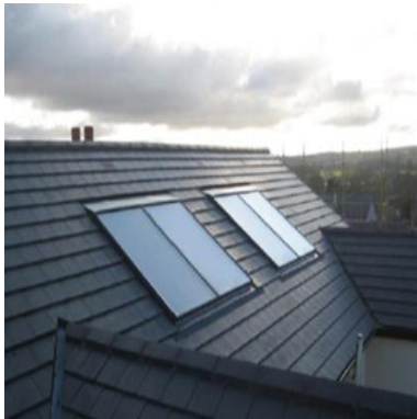
Figure 2.4. Roof integrated flat plate BISTS
