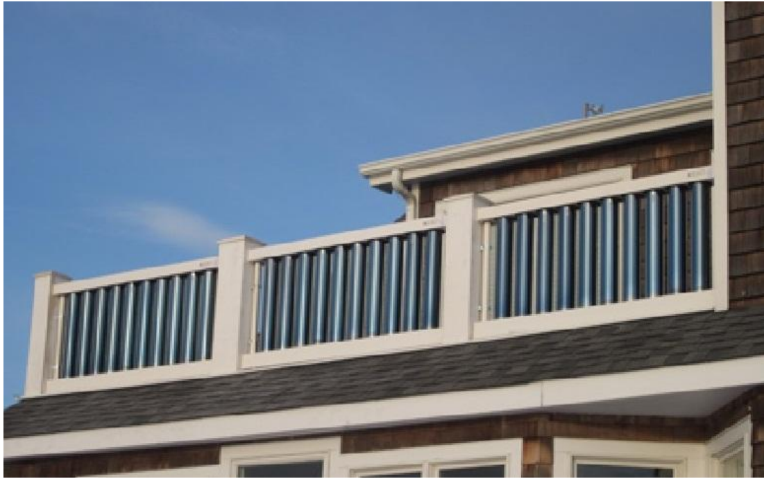
Figure 2.18 The JET Solar Fence (JSF) installed in a domestic building in USA.
